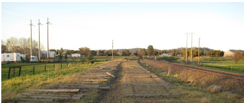
North end of proposed South Cowra intermodal terminal site
