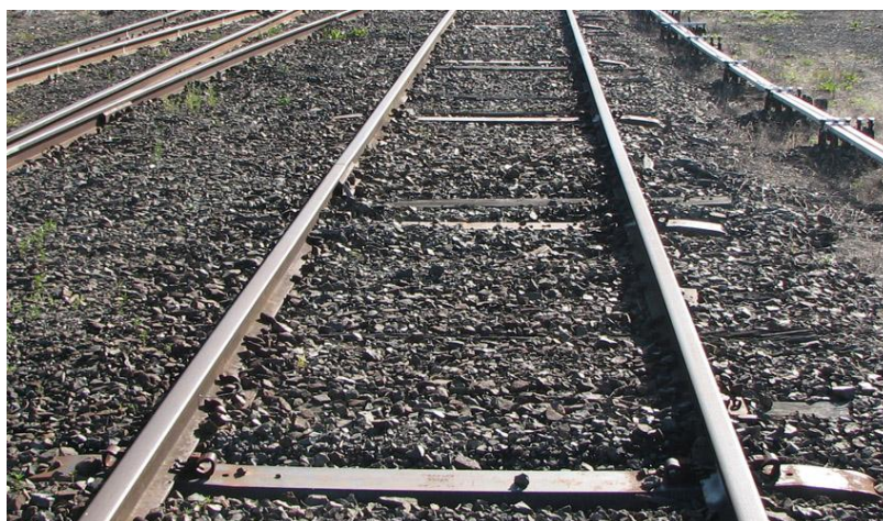
Track with mixed steel and timber sleepers
