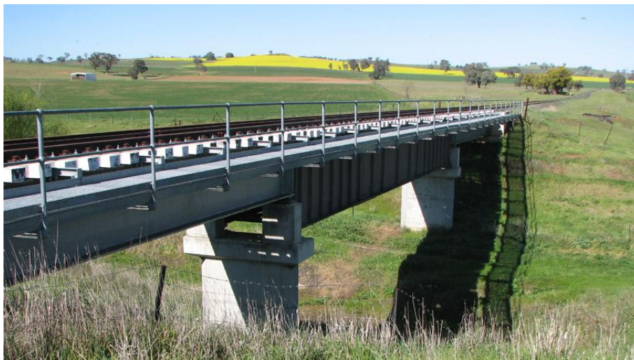
Rebuilt Waugoola bridge
